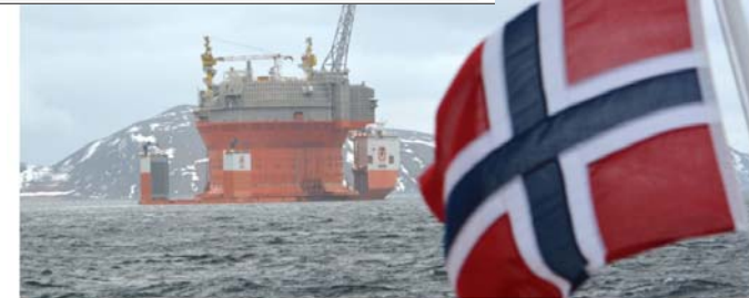
The Gullst platform was brought north in 2015 and became Norway's first oil production field in the Barents Sea. Photo: Thomas Nilsen
